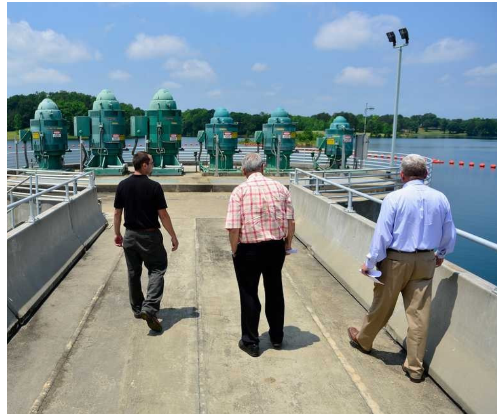
Bear Creek Regional Reservoir & Treatment Plant
