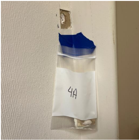
4A, Wall System, Meeting Room Connected to Printing Area
