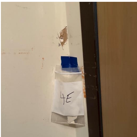
4E, Wall System, Electrical Room
