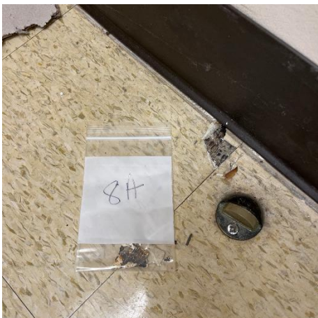
8A, Tile, Wheelchair Storage Room
