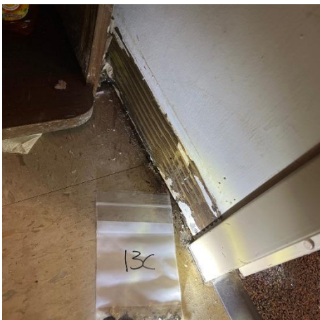
13C, Cove Base Adhesive, Water Heater Room
