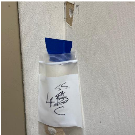
4C, Wall System, Wheelchair Storage
