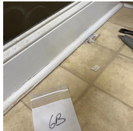
6B, Tile, Center Hall Men's Bathroom
