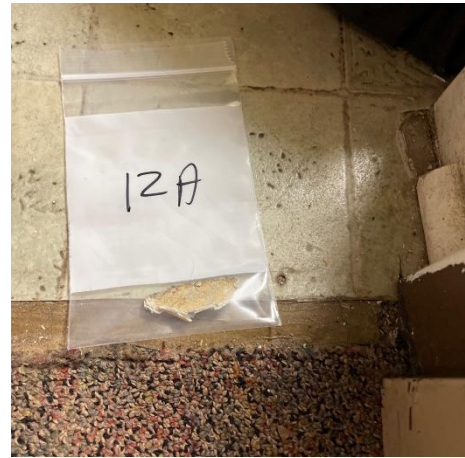
12A, Resilient Floor Covering, Women's Restroom
