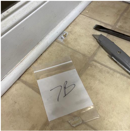
7B, Resilient Floor Covering, Center Hall Men's Bathroom
