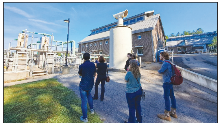
NEGRC staff look at step 1 of the Cedar Creek Water Reclamation Facility treatment process, receiving the wastewater and removing solids.
