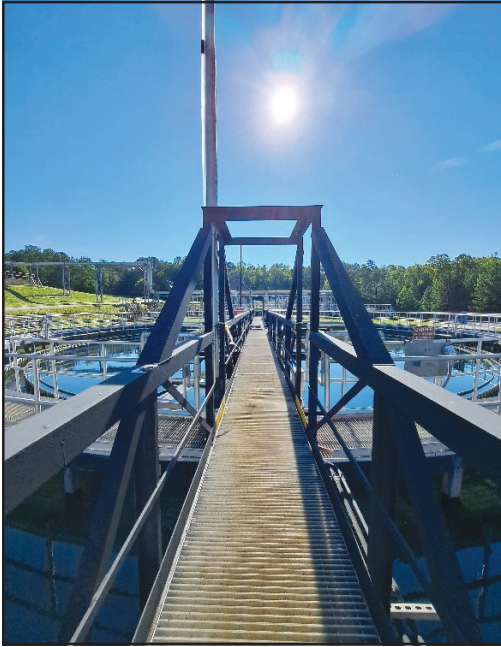
View above the final sedimentation tank. An agent is used to coagulate microbes and other biomaterial to be removed from the water. Water is then sent through UV treatment before being discharged into the Oconee River.
