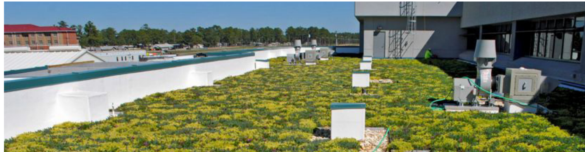
Example of a green roof at the Federal Army Hospital at Fort Stewart, GA
