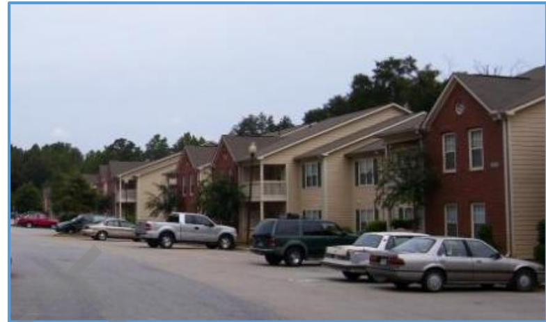
Example of apartment units in Commerce that are part of the urban residential character area.
