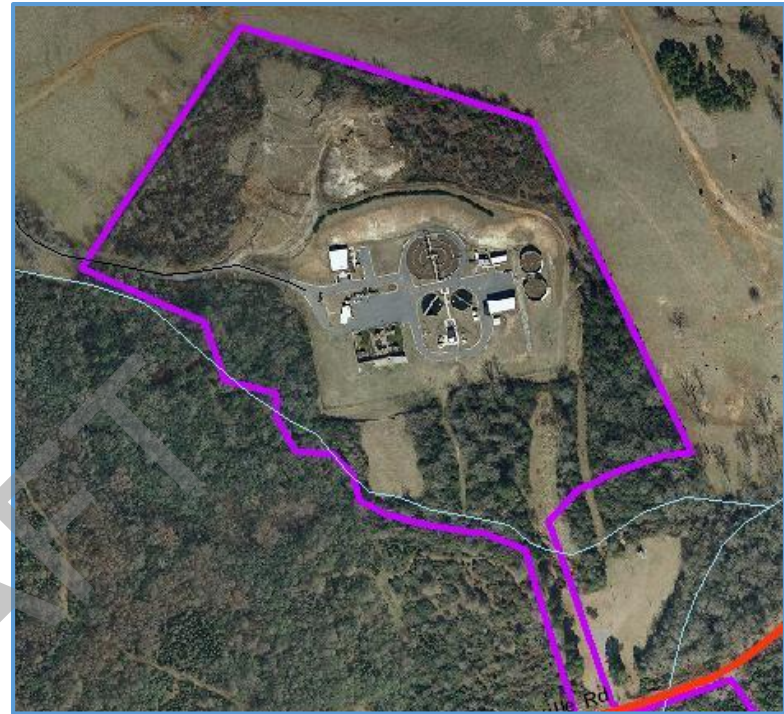
Commerce's treatment plant is an example of a special, single-use character area.
