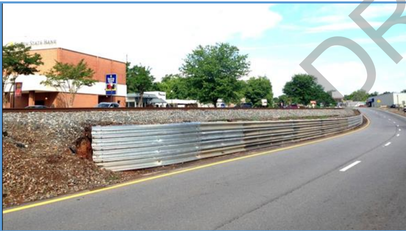
Retaining wall repair on Broad St.
