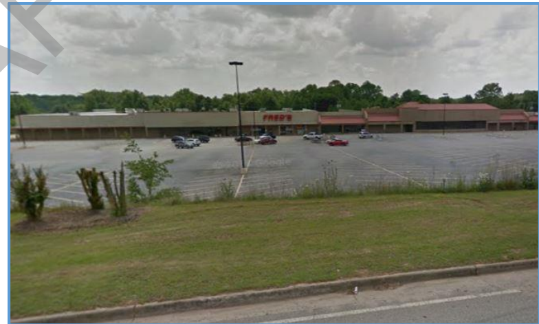
This largely vacant shopping center is along a major gateway corridor coming into downtown.
